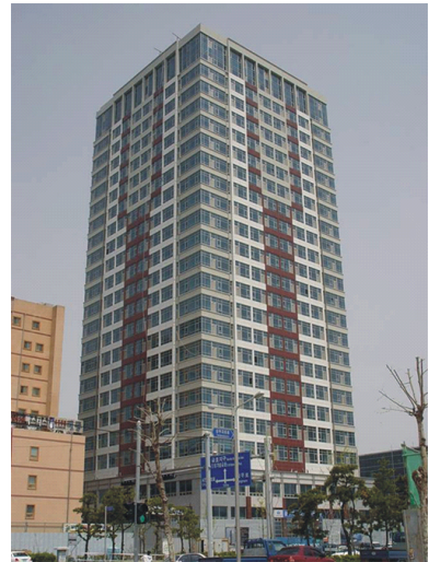
(a) Overall view
