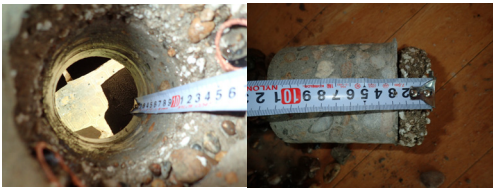
Fig. 1 Floor boring scene
