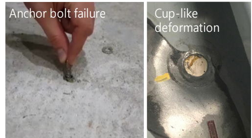
Fig. 7 Anchor bolt failure and local deformation after test 11 (200%)
