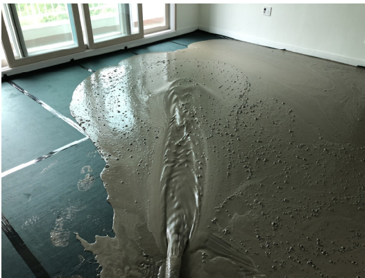
Fig. 2 View of installing the specimen
