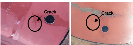
Fig. 8 Crack on the rope guard
