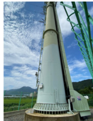
Fig. 1 High-voltage TST field test
