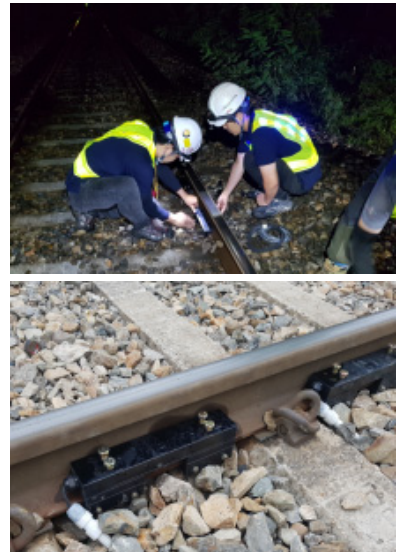
Fig. 9 Rail sensor installation
