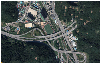
(a) Aerial image
