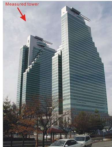
(a) Overall view
