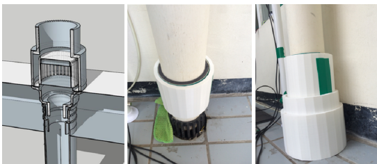
Fig. 4 Drain cover 3D modeling and applied drain cover
