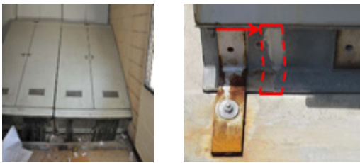
Fig. 1 Type of damage to operating facilities
