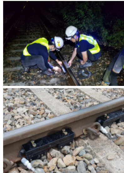
Fig. 9 Rail sensor installation
