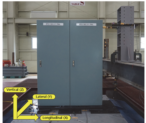
Fig. 2 RTU panel with non-overtum seismic isolator on the shaking table
