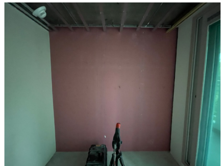
Fig. 2 Test specimen installed in mock-up house
