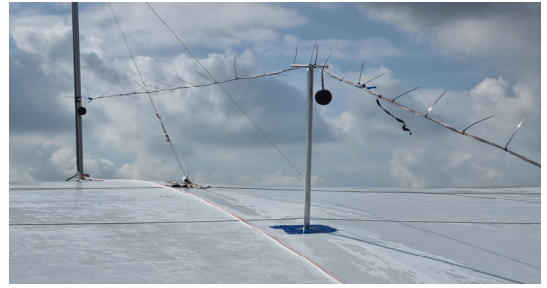
Fig. 7 Microphones installed outside of the soundproof tunnel
