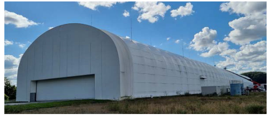
Fig. 5 Mock-up of the soundproof tunnel with membrane material
