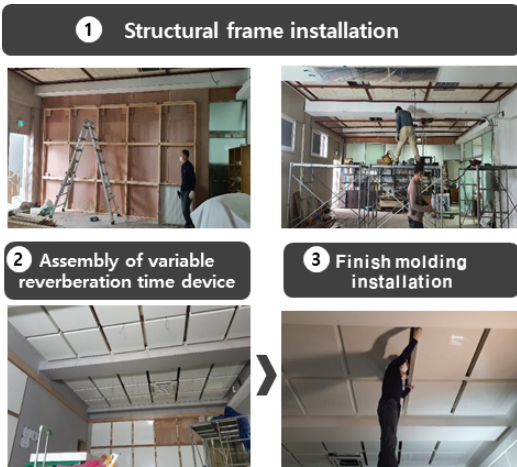
Fig. 5 Installation photo of the developed reverberation variable device
