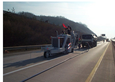
(c) Under construction
