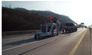
(c) Under construction
