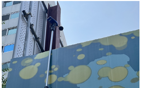
Fig. 6 Noise monitoring equipment installed at construction site A
