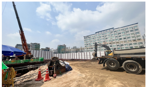
Fig. 7 Construction equipment position within the construction site A
