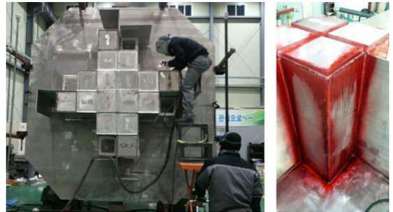
Fig. 11 Stiffener welding and liquid penetrant examination
