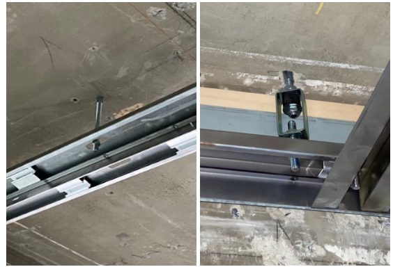
(a) Hanger (b) Anti-vibration hanger
