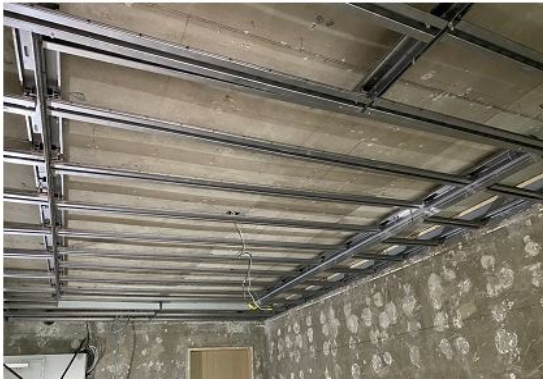
Fig. 2 Installation of the ceiling structure in receiving room
