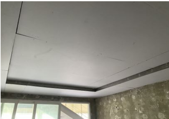
Fig. 3 Tray ceiling finished with gypsum boards
