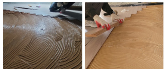
Fig. 3 Installation of epoxy adhesive (left), and poly-urethane-based adhesive (right)
