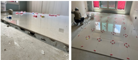
Fig. 6 Installation of floor tile adhesive
